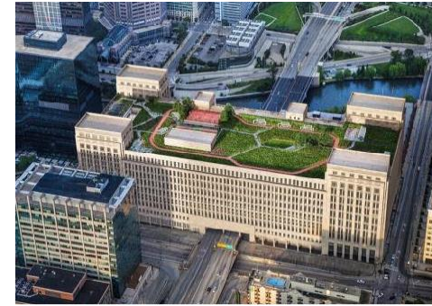
Old Post Office Chicago Two million square ft. installation in Chicago (2019)
