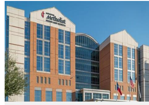
METHODIST HOSPITAL (TX) AtmosAir helped reduced major sewer gas odors and improve perceptual air quality.
